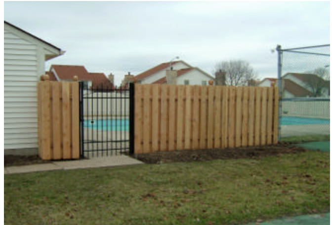
New front gate fence was installed in January in time for the Memorial day opening. The board hopes this will give our residents more privacy and prevent non-residents from using our pool. Please contact our association managers for a new key.
